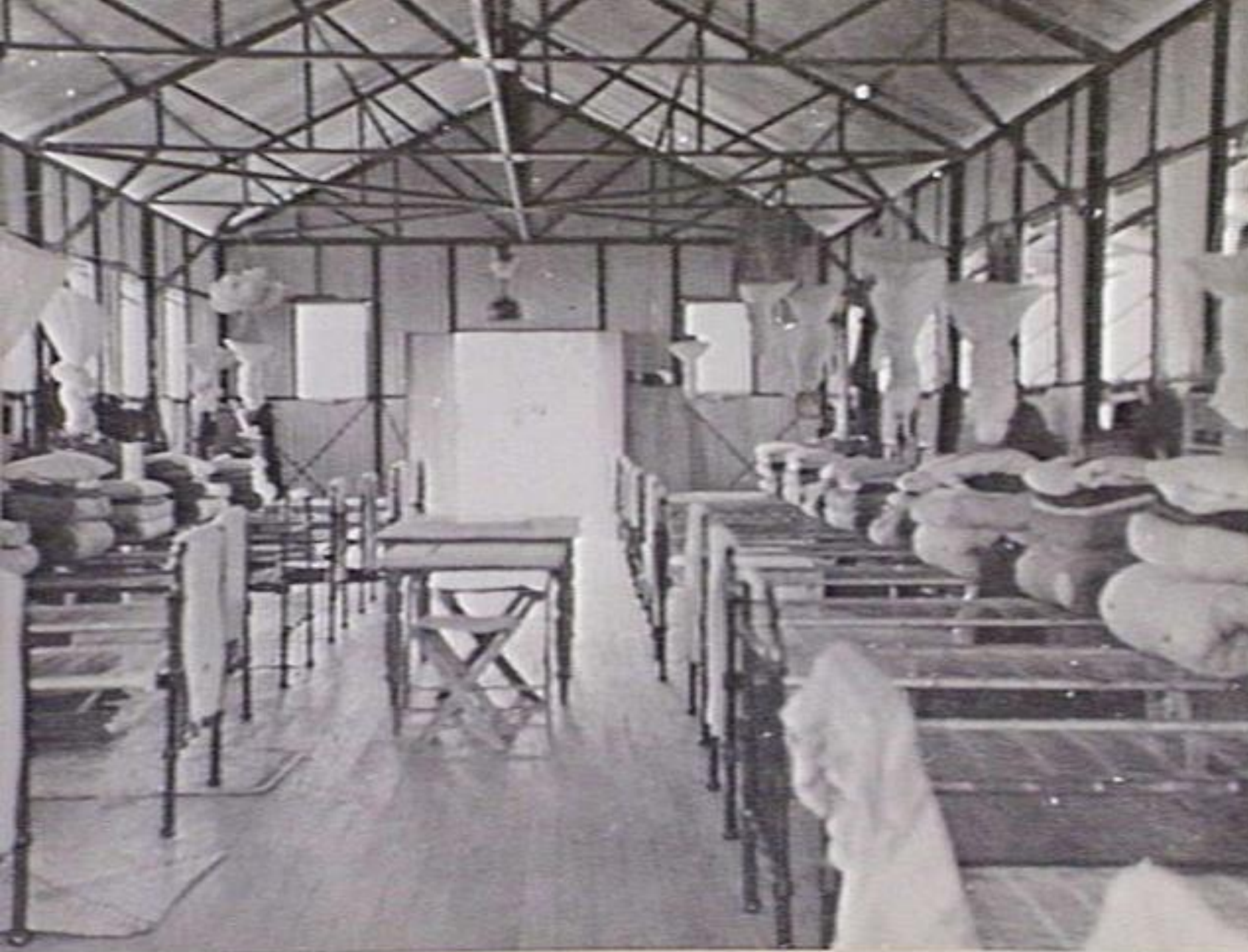
PORT MORSEBY, PAPUA. INTERIOR OF A NEWLY CONSTRUCTED RAAF BARRACKS AT KONEDOBU CAMP. (PHOTOGRAPHER N. J. TRACEY )
