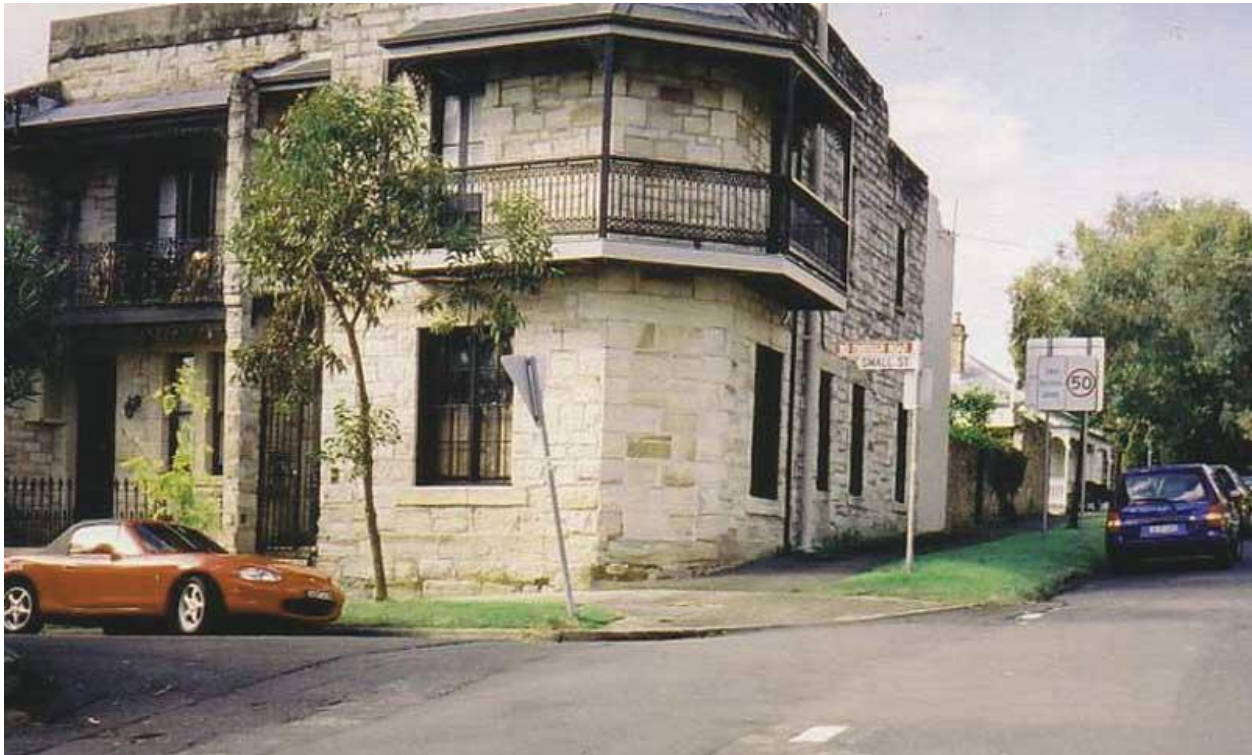
The bombed shop on the corner of Small and Fletcher Streets, Woollahra
