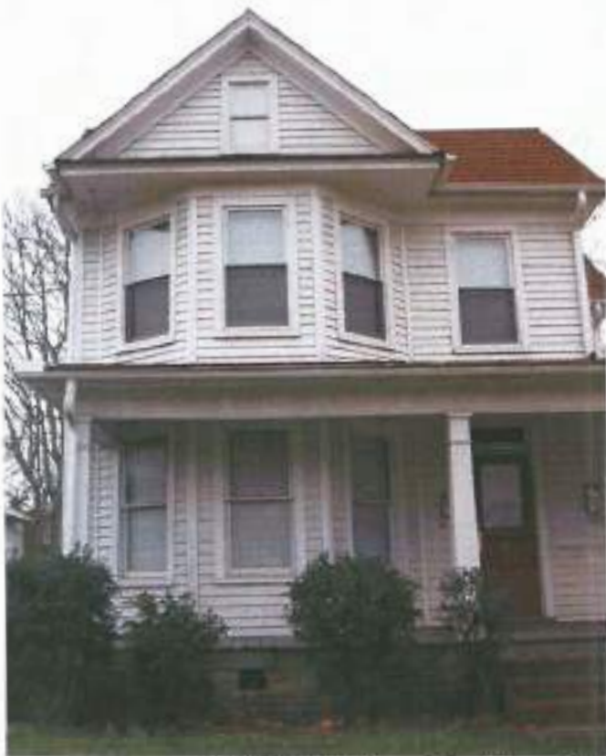
The house at 1202 Stewart Street has the gable-and-wing form.
