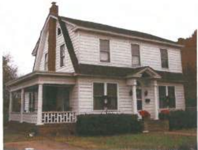
At 1138 Chesapeake Avenue is a Dutch Colonial Revival house. The most distinguishing feature of this type of Colonial Revival building is its gambrel roof. Often Dutch Colonial Revival houses have large shed dormers, as shown here.
