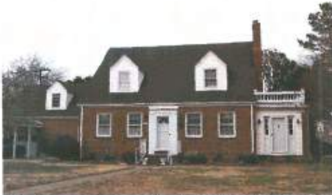
The dormers, side-gabled roof, classical-inspired entry surround, and symmetrical façade on the house at 1201 Orville Avenue are all Colonial Revival features.
