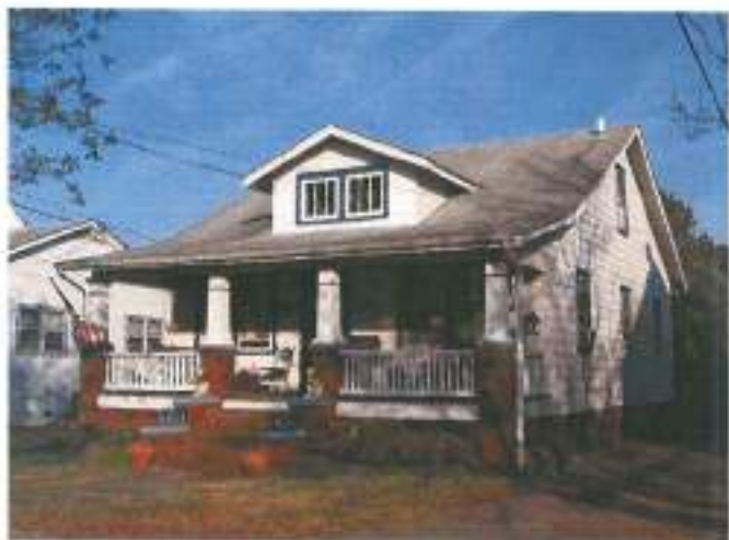
The Bungalow at 1321 Jackson Avenue has many Craftsman features, including the tapered wood posts above brick piers that extend to the ground and the full-width porch.
