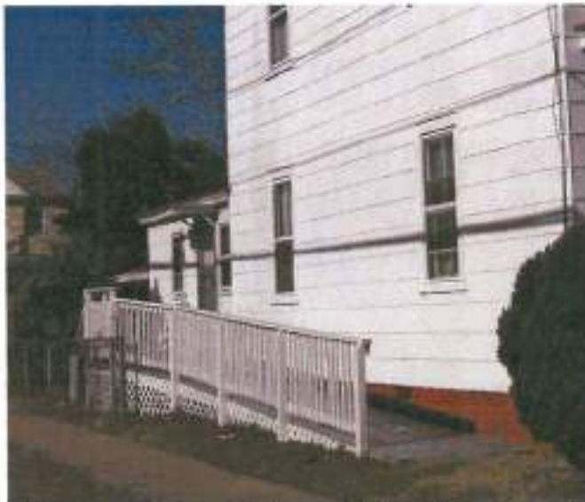
The ramp on 1232 Stewart Street is appropriately placed and painted.
