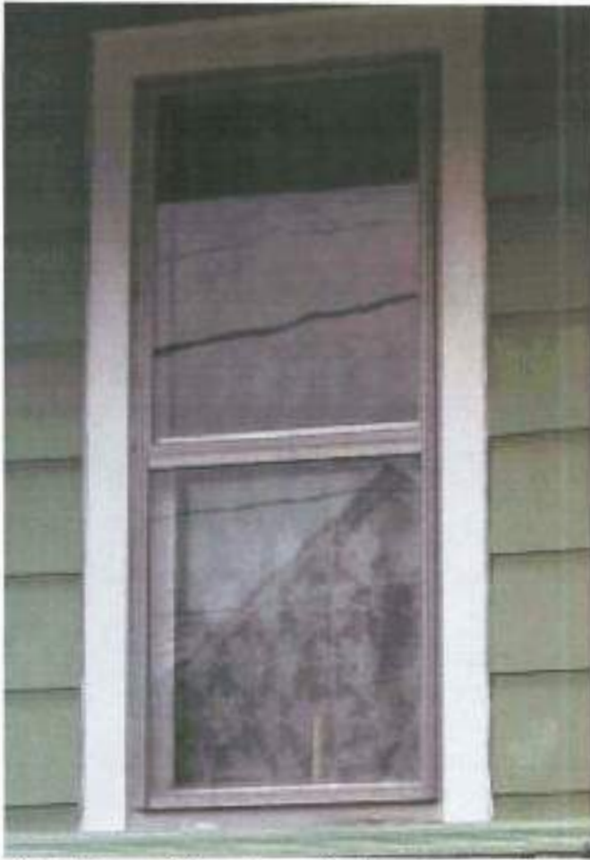
The design of the storm window at 1332 Chesapeake Avenue, with a central meeting rail in the same place as the window's, is appropriate.
