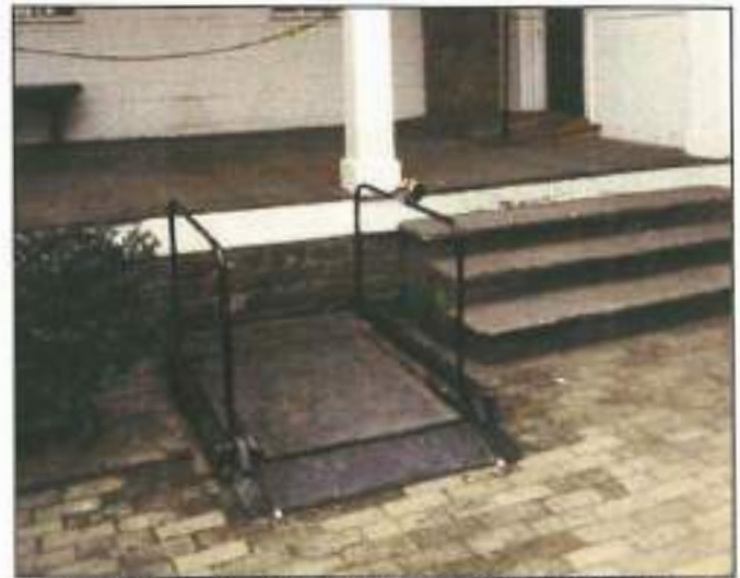
Wheelchair lifts, ideally placed along side or rear elevations, may also be helpful for accessibility.
