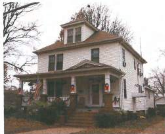
The American Foursquare, square buildings with hipped roofs, became a popular house type around the turn of the twentieth century. In South Norfolk, this type is also called Square Hipped. American Foursquares were often built with Prairie, Craftsman, or, as at 11238 Chesapeake Avenue, Colonial Revival influences. Their simple forms blended well with the conservative Colonial Revival aesthetic.
