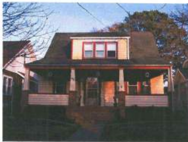
The shingles on the dormer at 1321 Rodgers Street reflect a Craftsman interest in materials and textures. Other Craftsman features on this Bungalow include the exposed rafter tails below the dormer eave, the three-over-one dormer windows, and the tapered wood posts on brick piers.
