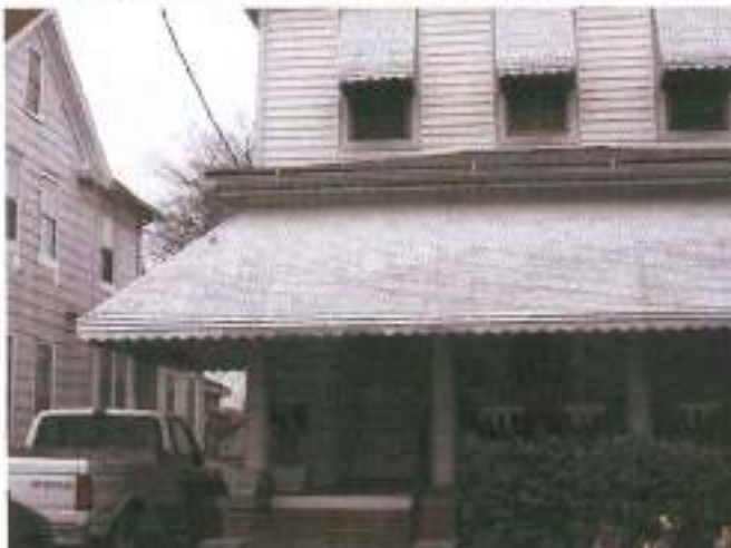
The historic metal awning on 1309 Chesapeake Avenue and others like it should be retained and kept in good repair.
