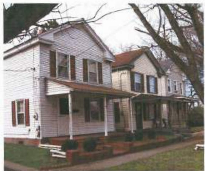
The front-gable form was a popular one, and rows like this one on the 1100 block of Hoover Avenue are common.
