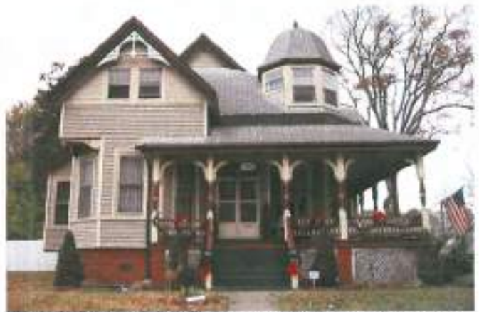
The complex roofline, tower, varied projections, one-story porch, and trim on the house at 1106 Chesapeake Avenue are all Queen Anne features.
