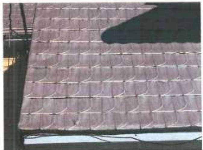
Gentle cleaning methods can prevent damage to metal components like the shingles on 1221 Park Avenue.
