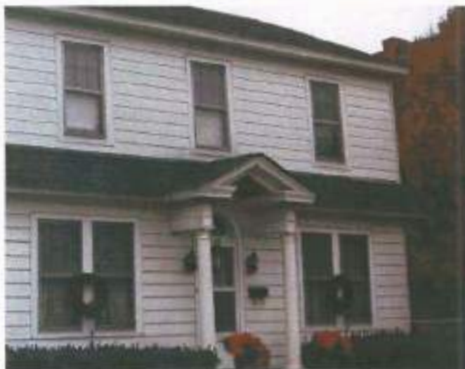
Existing synthetic siding may be replaced with new synthetic siding materials (1138 Chesapeake Avenue).
