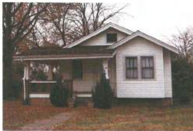
Repeated front gables, like those on the house at 1132 Decatur Street, were popularly used on Bungalows. Multiple-pane-over-single-pane windows like those shown here are common Craftsman features.
