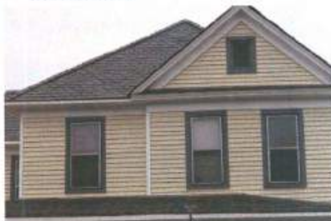
Paint helps protect wooden elements like the wood siding on 1238 Chesapeake Avenue from decay.
