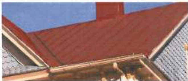
Historically painted metal roofs like the one on 1041 Chesapeake Avenue and other surfaces should remain painted.
