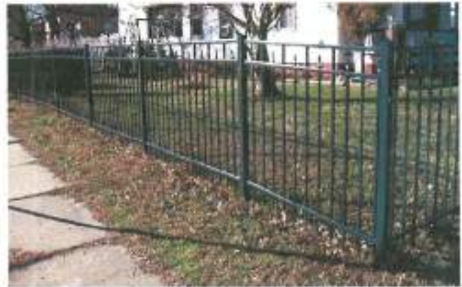
This simple metal fence at 1236 Seaboard Avenue uses materials, design, and color appropriate for its historic setting.
