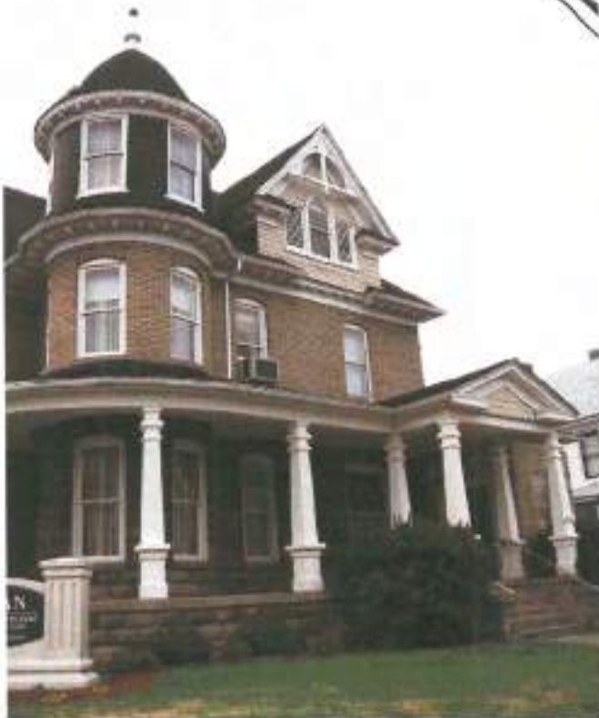
The Queen Anne house at 1146 Rodgers Street has many typical Queen Anne features: multiple surface treatments, a tower, a wrap-around porch, trim work, and bays with various levels of projection.
