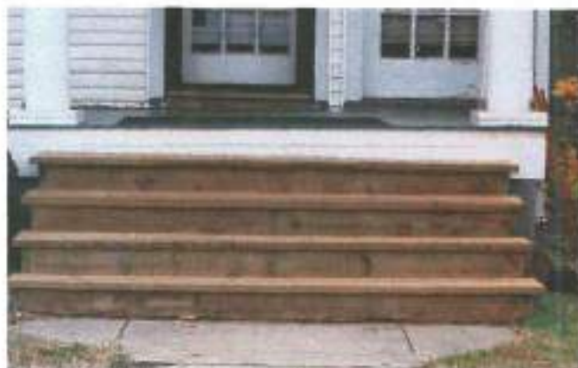
These replacement porch stairs at 1326 Chesapeake Avenue appropriately used wood to match the wooden porch.
