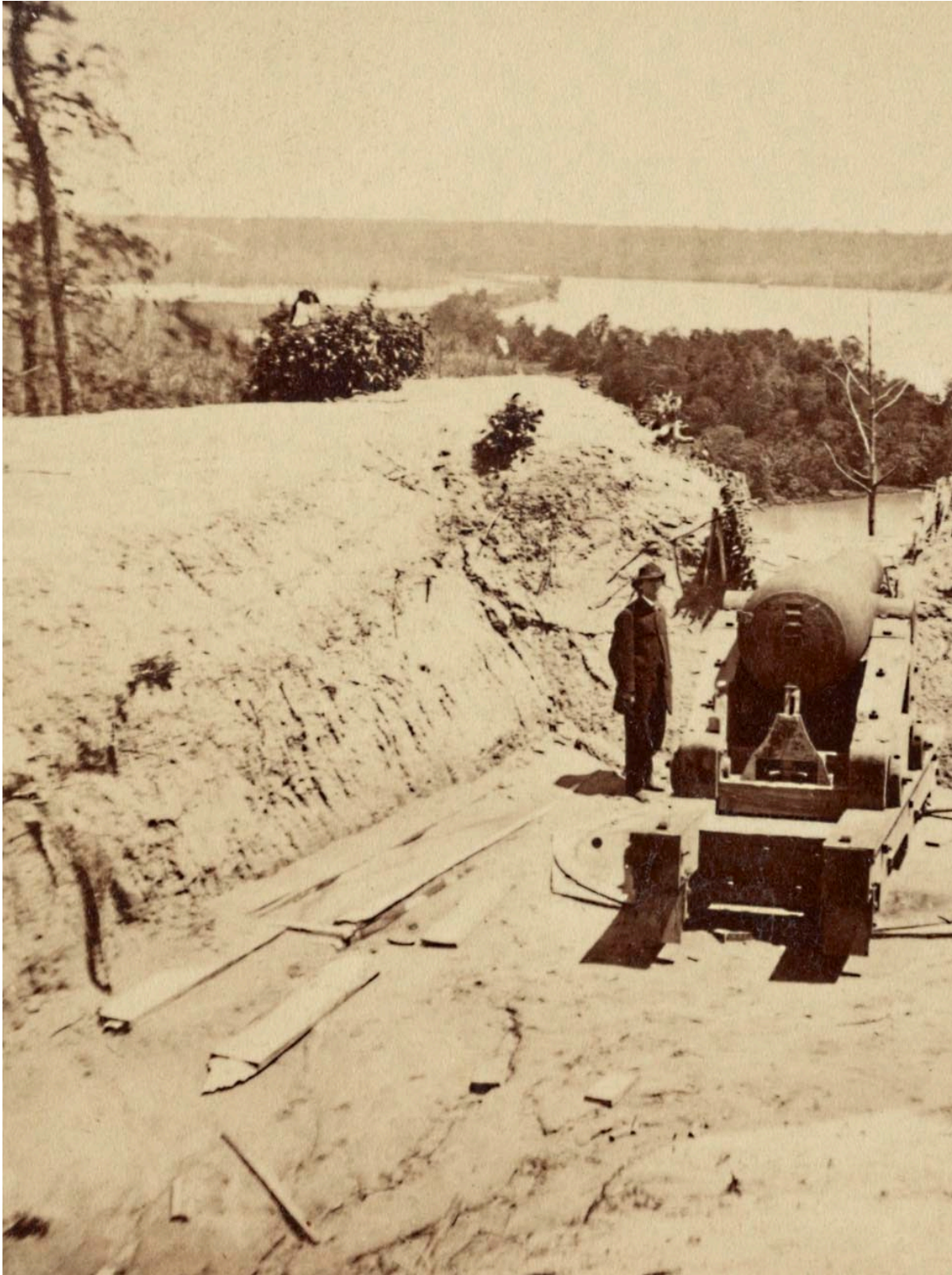
One of the 10-inch Columbiads at what was known by the Confederates as Battery Dantzler overlooks the James River in this image taken after its abandonment in April 1865. Cmdr. William A. Parker's concern over the two Columbiads and two Brooke rifles overlooking the James about three-quarters of a mile above Trent's Reach at what he called "Howlett's Battery" prompted a cautious approach. ( Civilwartalk.com )
